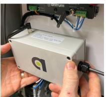
Slide the sensor pack to the right while positioning the ¼" tubing to align with the bulkhead fitting(s). Using gentle pressure, insert the ¼" tubing into the fitting(s).
